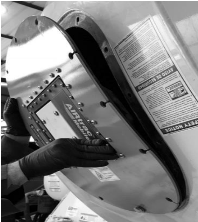
Figure 9: SMARThatch Sensor Lifted into Position
